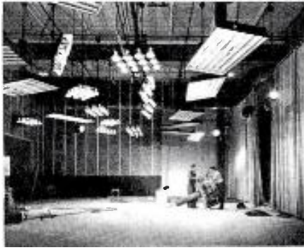
Studio A, 60'x 40', is equipped with 39 suspended lighting fixtures... permits simultaneous display of 8 automobiles on one set.
