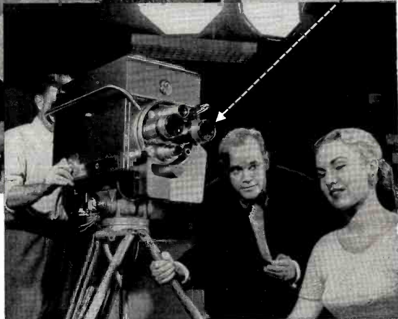
▲ G-E camera above is ready for color. Note close similarity in size to the monochrome unit left above.
